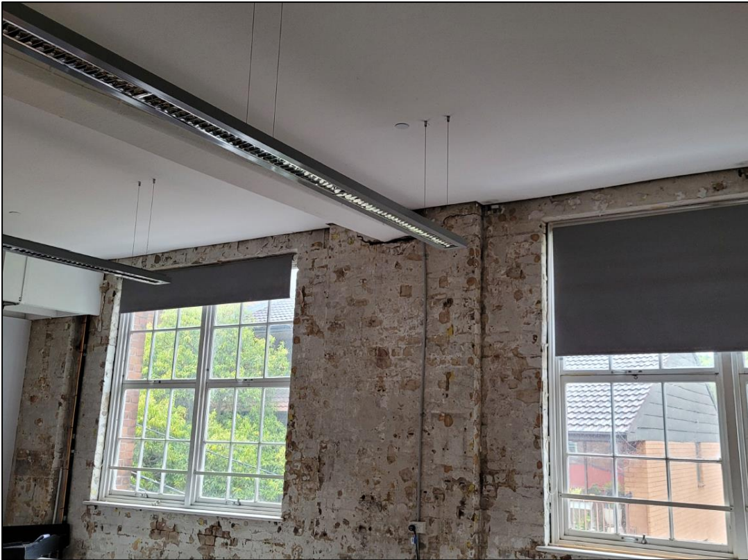
Figure 9: Existing south facing windows on Level 3
