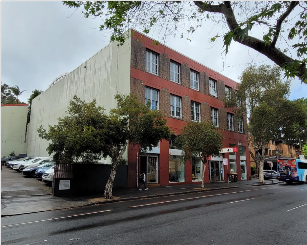
Figure 5: Site viewed from Elizabeth St looking south-east
