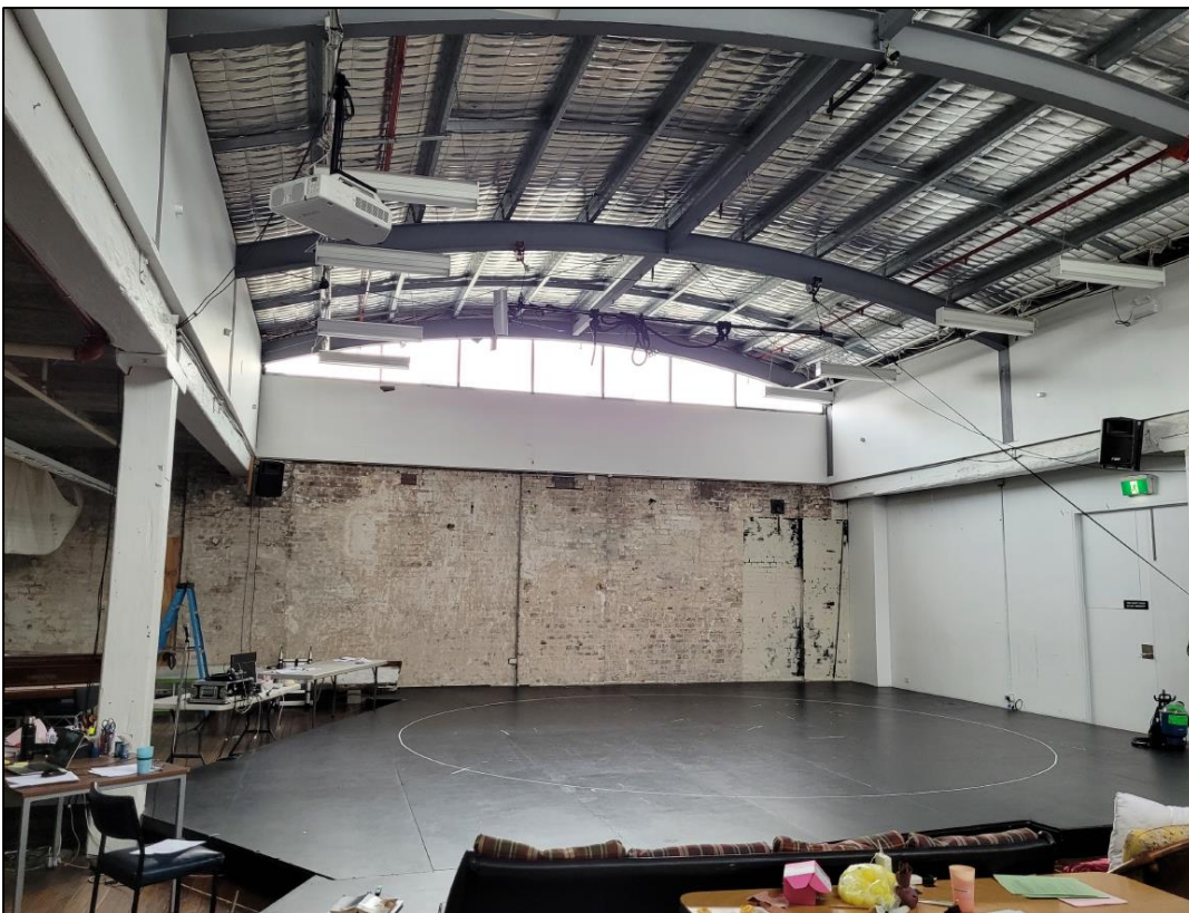
Figure 8: Internal view of the Belvoir Theatre company rehearsal space on Level 3
