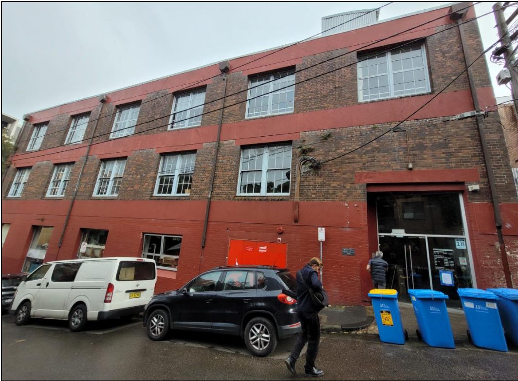
Figure 3: Site viewed from Belvoir Street
